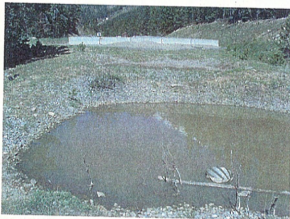
3 Sedimentation: CDOT sediment retention ponds at Herman Gulch.
