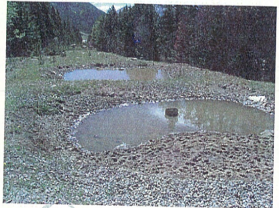
2 Sedimentation: CDOT sediment retention ponds at Herman Gulch.
